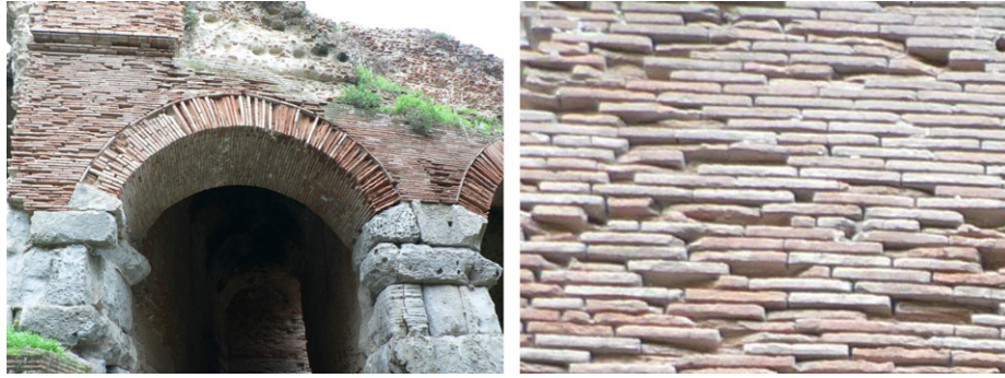
Fig. 4. An example of Roman masonry (Anfiteatro Flavio, built in the second half of the first century A.D. under Emperor Vespasiano at Pozzuoli, Naples. Photo by D. Bigoni). A detail is shown at right of the masonry in the upper left part of the figure at left.
