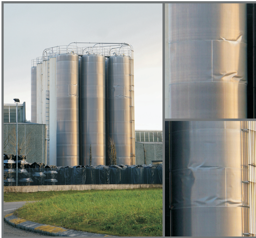
Figure 24. Local buckling in two silos (near Bazzano, Italy).
